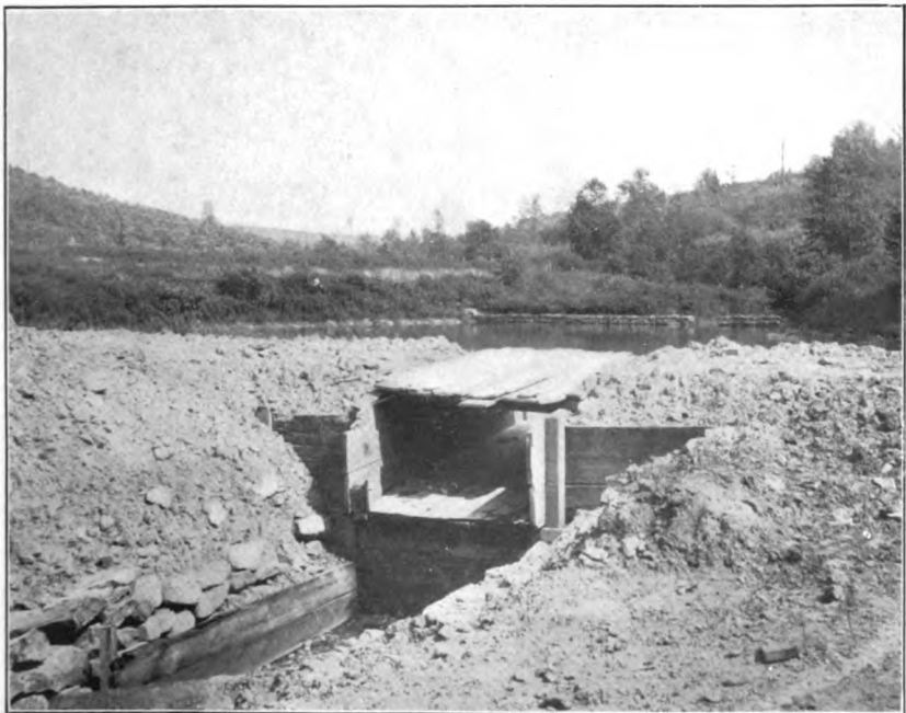
B. DAM AND RESERVOIR OF PUBLIC SUPPLY AT REYNOLDSVILLE PA.
